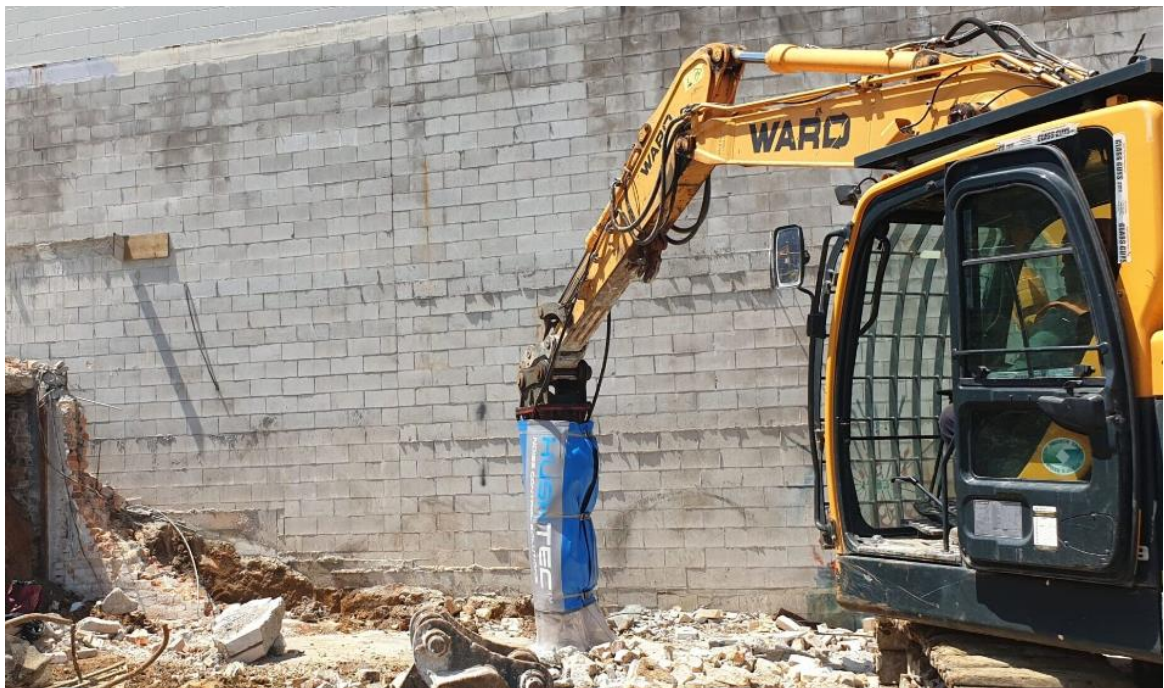
Figure 4: Rock breaker shroud
